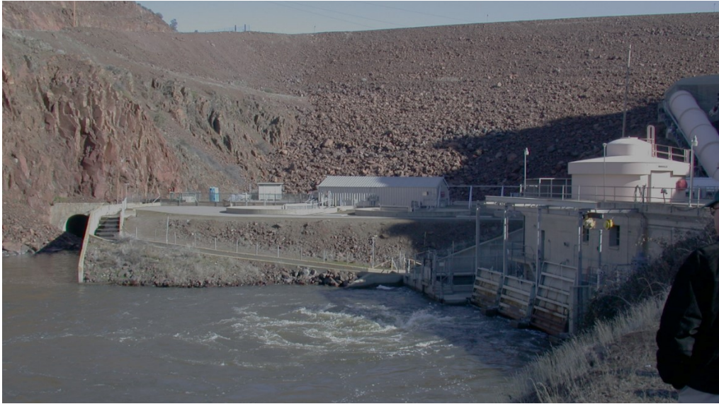
The foot of Iron Gate Dam, located 190 miles upriver from the mouth of the Klamath. To the left is the emergency drain tunnel (never used). Left center is a fish ladder that leads to a collection facility for the hatchery. To the right is an electric generation turbine that is fed by the penstock pipe in the far right background.
