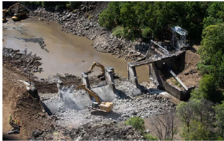
Dam removal begins.
