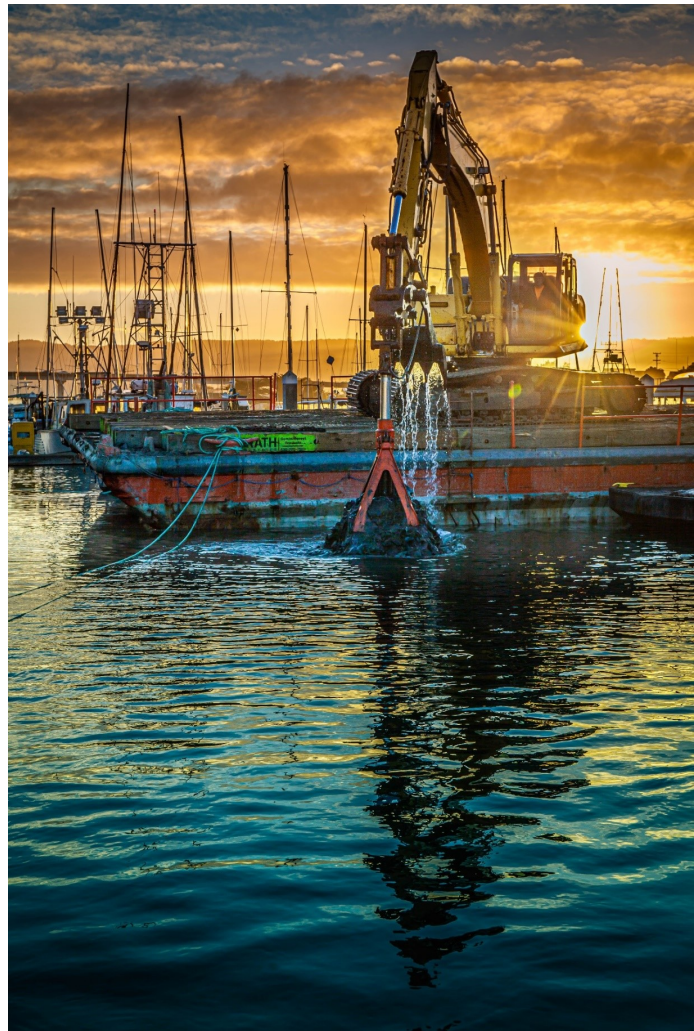
2020 Dredging in Woodley Island Marina.
