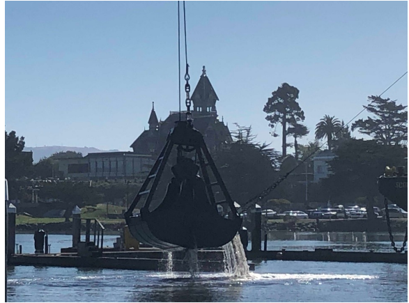
Clamshell bucket removing sediment at Woodley Island Marina.
